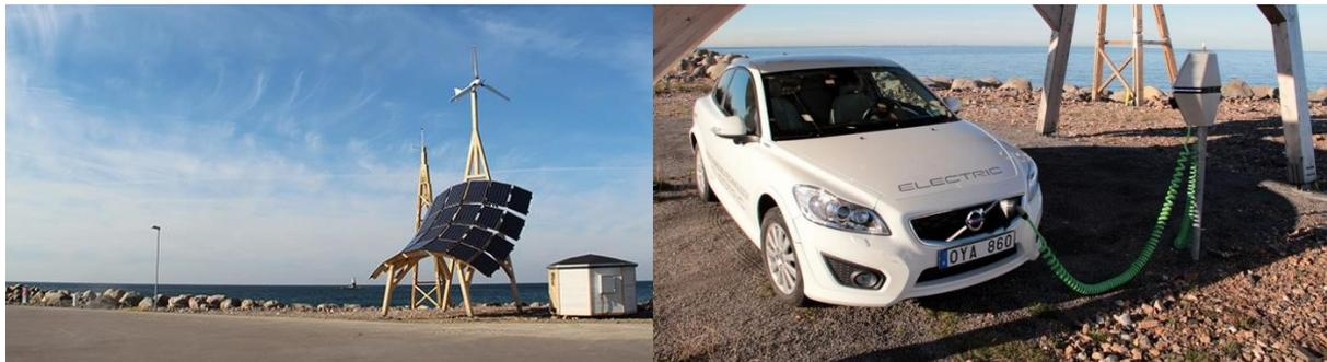
The Giraffe is designed to protect two cars and covers a total area of two parking spaces. In other words, there is no loss in parking space when installing Giraffes that are delivered with a double-quick-charger from Chargestorm that gives 2 x 22.1 kW via 32 A 400 V.
